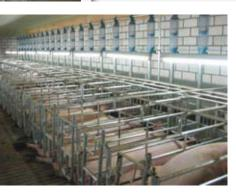
fattener houses. In all the houses a ventilation ceiling is made of perforated sheets and glass wool. Climate of each room is separately controlled by means of control panel.
